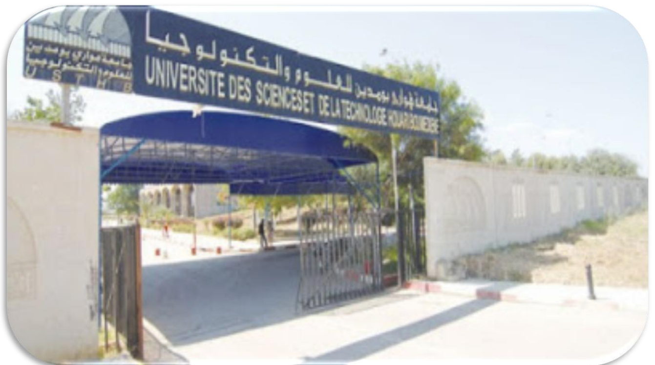
Entrée principale (cloture)
