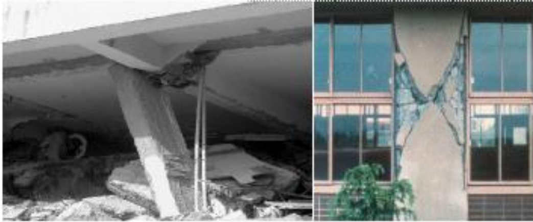
Figure I.9: cisaillement des poteaux courts.
