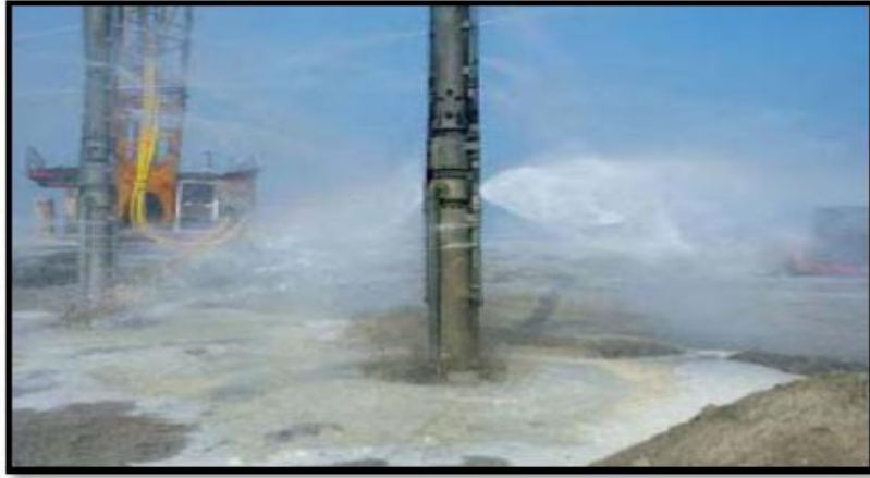
Figure III.5. Vibrocompactage. (Kazi Aoul, 2015).
