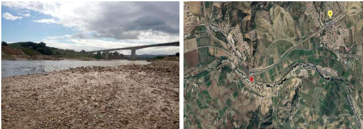
Figure 11. Station de Tadmaït MS1.
