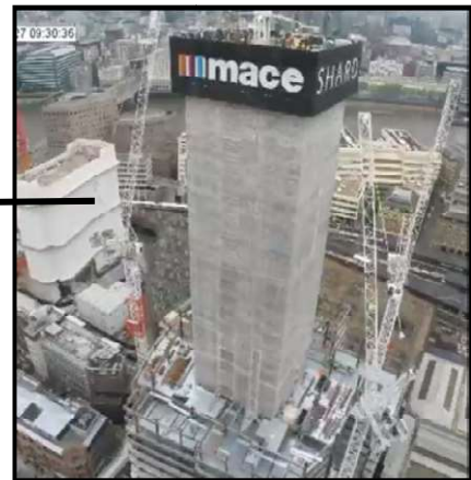
Figure 94: Le noyau en béton / Source: https://en.wikiarquitectura.com
