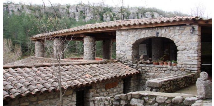
Figure 69: Le bâti village Source: France 5 (reportage)
