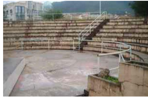
Figure 87:Amphitheatre Source: Auteurs
