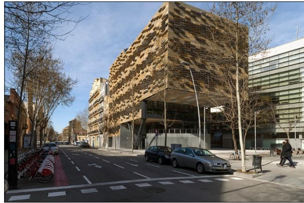
Figure 77 : Leitat Technology Center Source : Archdaily.com/776056/
