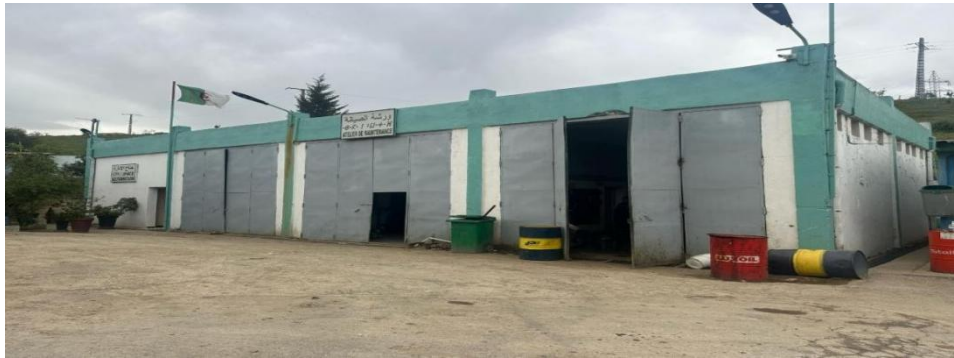
Figure 15: Atelier de maintenance (original,2025).
