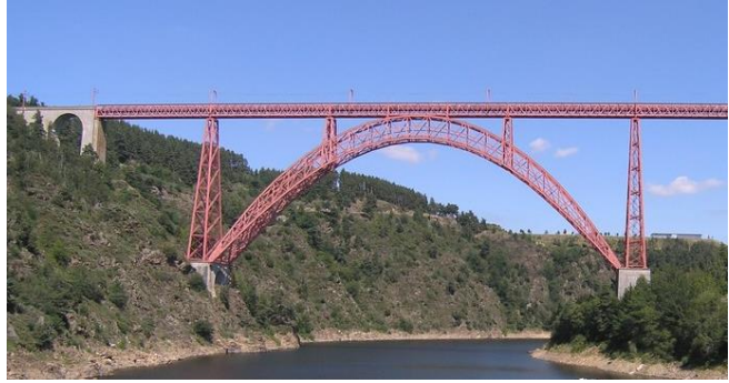
Figure I.12 - 1884 - G. Eifel & M. Kœchlin- le viaduc de Garabit – Garabit paris [8]
