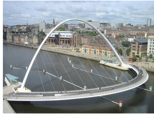
Figure I.18 -2001 -Brownlie – Gateshead Millennium Bridge – Londres [8]
