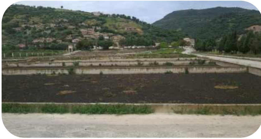
Figure 20: lits de séchage
