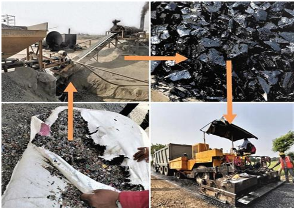
Figure I.11. Incorporating plastic waste into a road asphalt mixture. Source: ADB https://events.development.asia/
