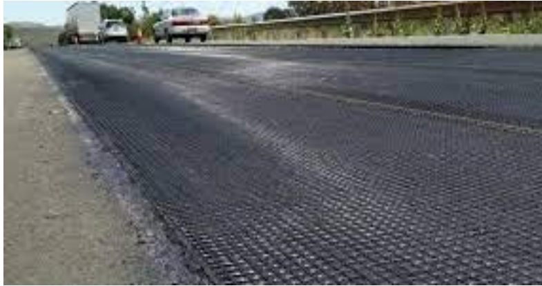
Figure I.10. Polyester fibers-based geotextiles in road construction usage. Source: https://oceangeosynthetics.com/importance-of-geotextile-in-road-construction/
