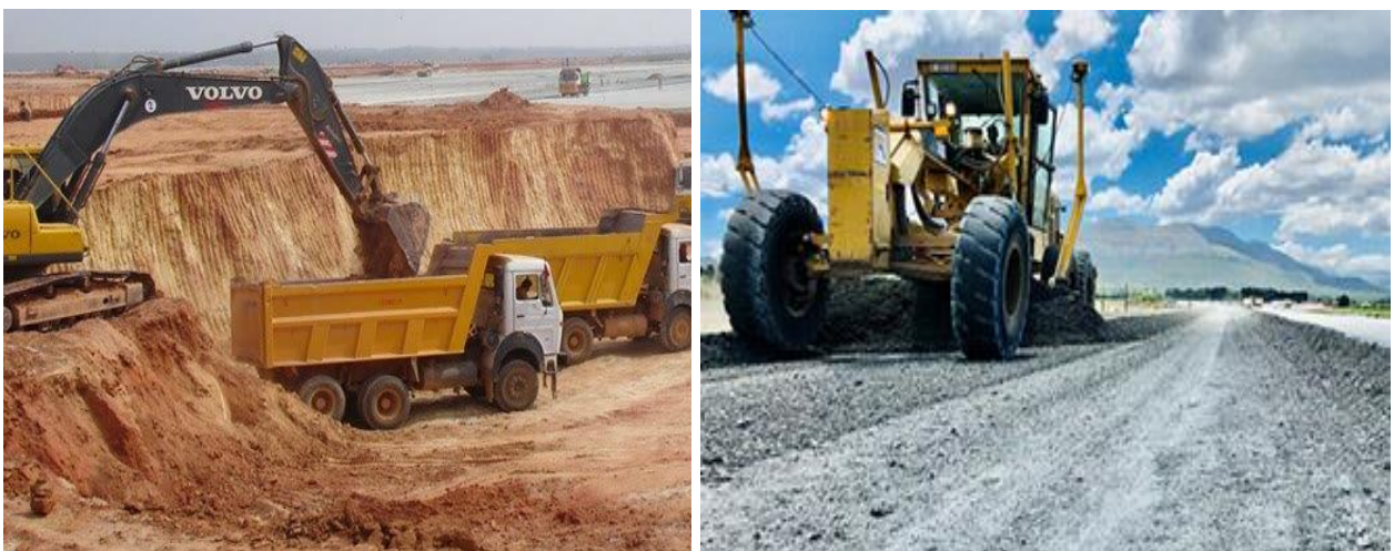
Figure V.5. Execution of embankment. Source: Indimart & Raubex https://www.indiamart.com/ & https://www.raubex.com/
