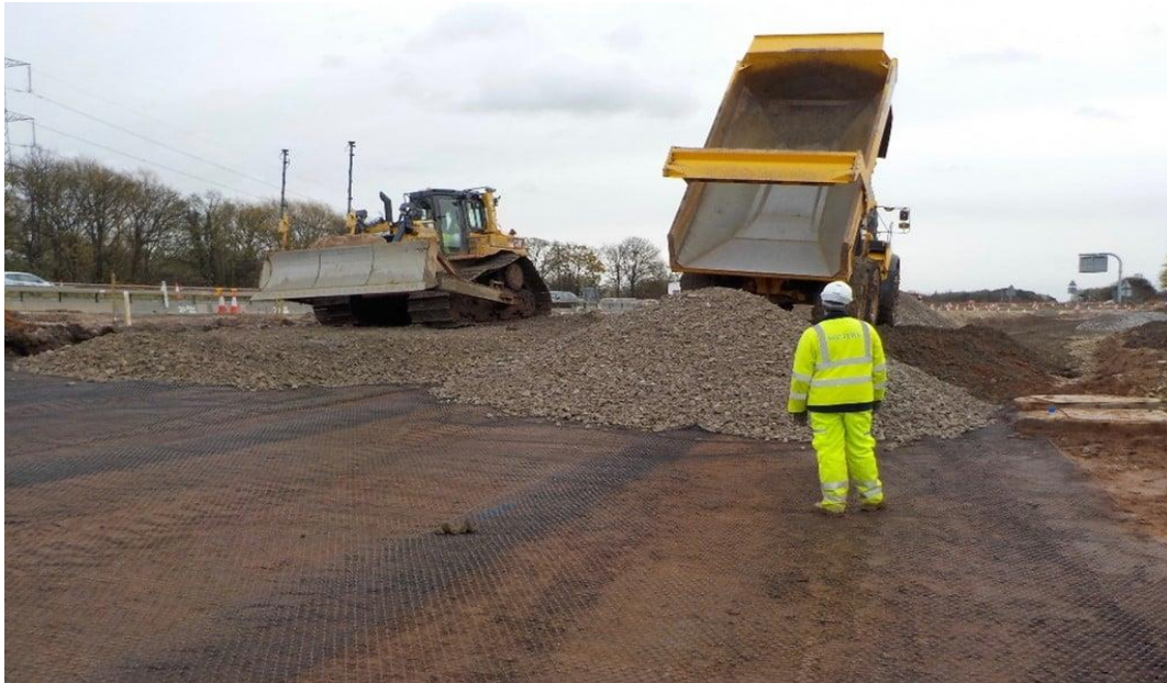
Figure V.6. Geotextile Installation and platform preparation. Source: Andrew Lees (2021) https://www.tensar.co.uk/resources/articles/what-are-the-different-types-of-road-construction-methods
