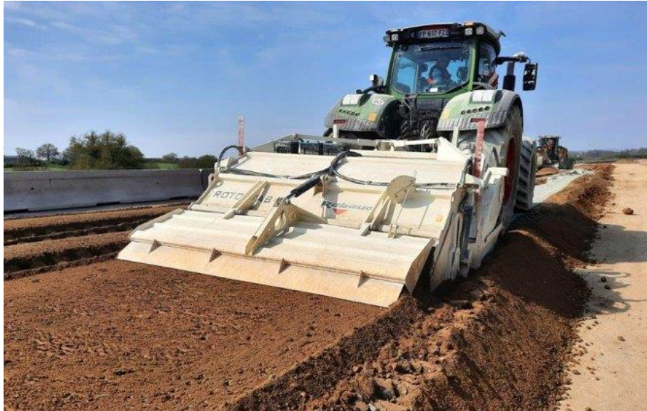
Figure V.12. Adjustment of the soil platform after compaction. Source: InfoCements https://www.infociments.fr/
