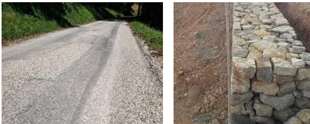
Figure I.7. Gravelly and stony materials used in road construction and protection. Source:
