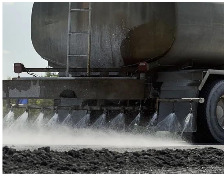
Figure V.13. Curing products application on the soil platform. Source: Eco Solution https://www.ecosolutiondistributing.com/coke-processing
