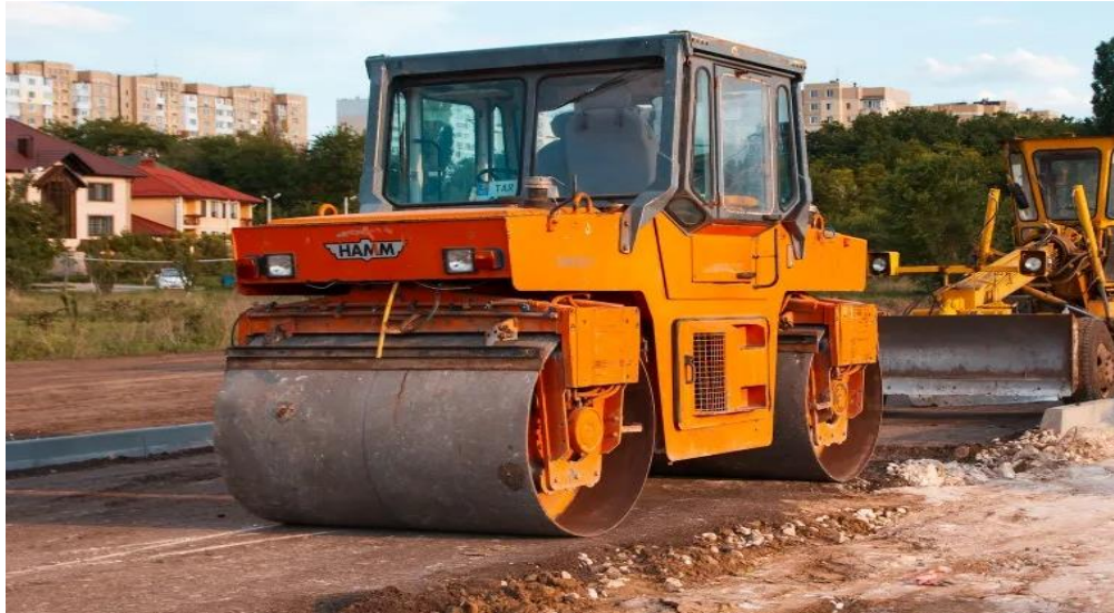
Figure V.11. Compaction of the soil platform after mixing. Source : Terra-Firma https://www.tfsoils.com/
