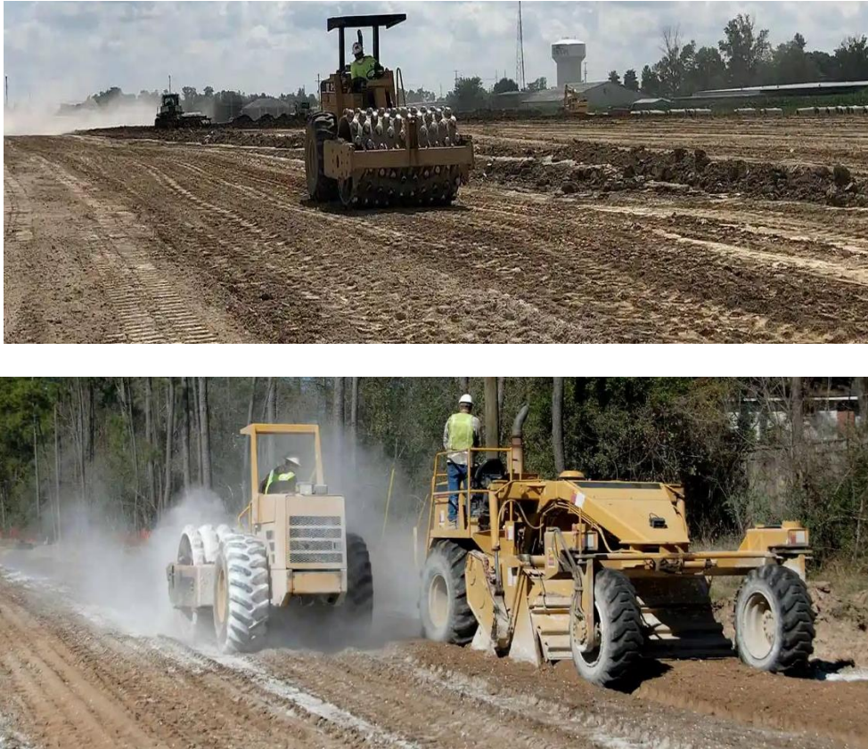
Figure V.10. Mixing of the soil after the binder application. Source: https://mintekresources.com/soil-stabilization-methods-and-materials/
