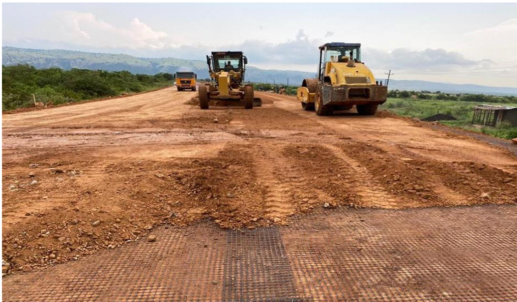
Figure V.7. Sub-base layer realization. Source : Admire Africa https://admirafrica.com/
