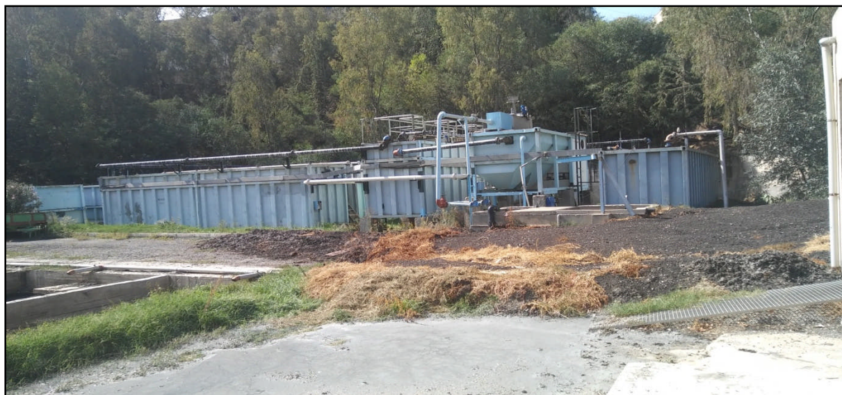
Figure 03: Ancienne station monobloc.
