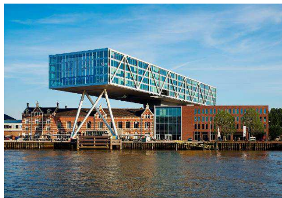
Figure 45 : Unilever Nederland BV. https://www.archdaily.com/261202/unilever-nederland-bv-jhk-architecten
