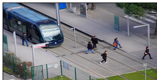
Figure 104: station de tramway interne Source https://operation-campus.u-bordeaux.fr/Agir-pour-un-campus-durable/Mobilite .
