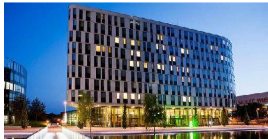
Figure 144 : Hôtel court yard Vienna mess.
