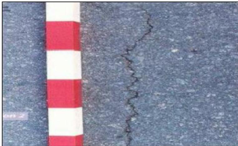
**Figure II.6. Fissuration transversale**
