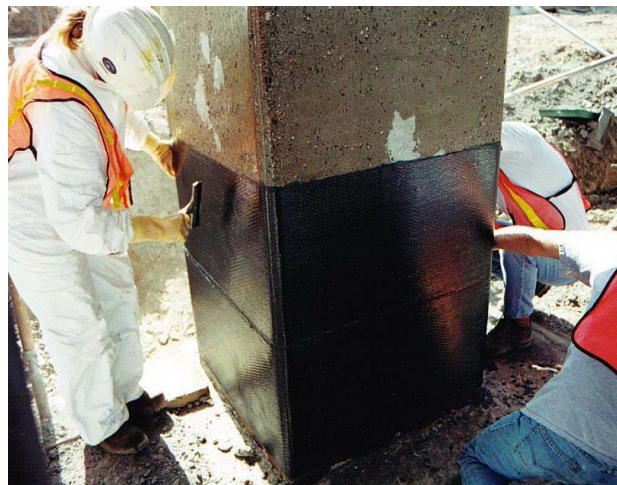
Figure III.18: Confinement de colonnes. [21]
