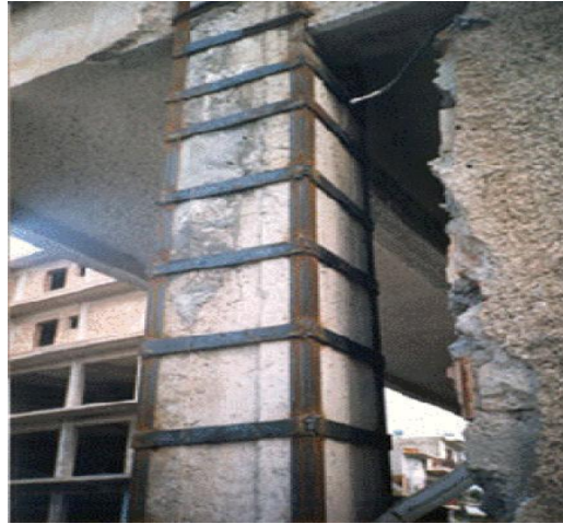
Figure III.2: Chemisage en acier [18]
