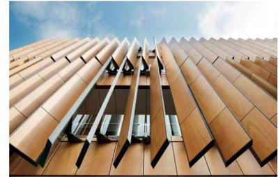
Figure III.41. brise soleil orientable
