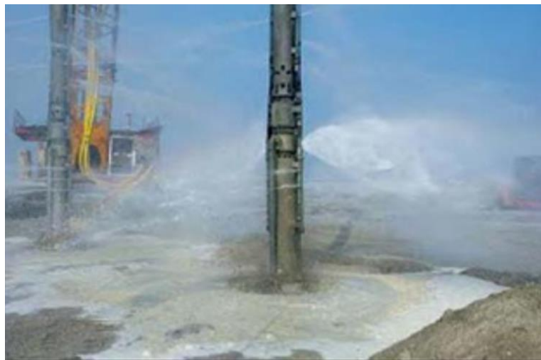
Figure II.2. Le Vibro-compactage.
