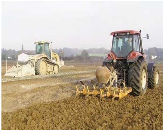
Figure II.16. Scarification des sols.
