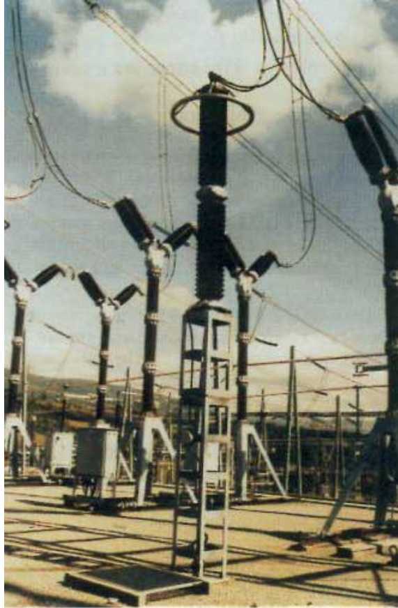
Figure II-11-B : parafoudre ZnO
