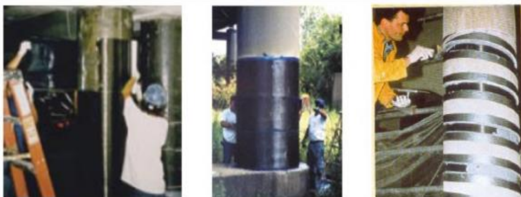
Figure II.15 : Stratification au contact (WBAC 2003) [43].
