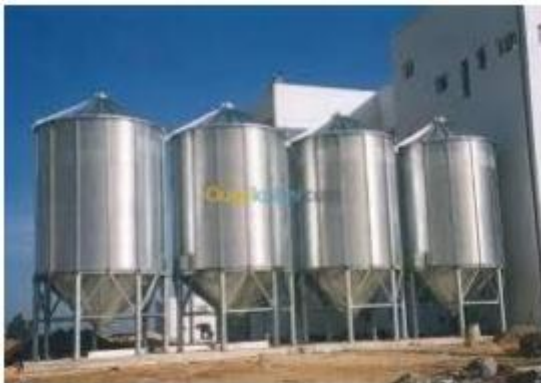
Figure 18: silos de stockage (ONAB)
