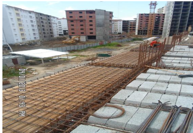
Figure I-3: Balcons en dalles pleines.
