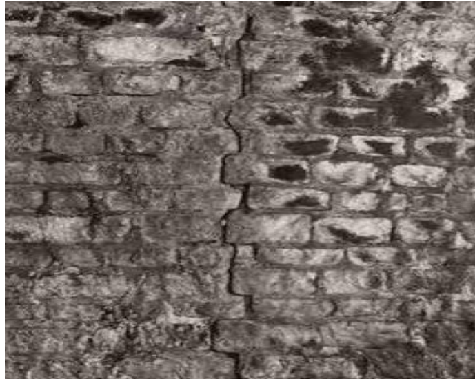
Figure II.11. Fissures transversales
