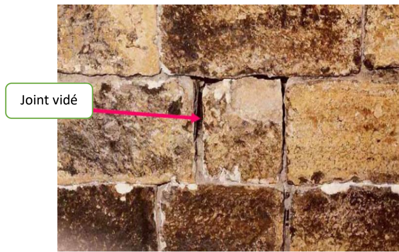
Figure II.8. Joints vidés
