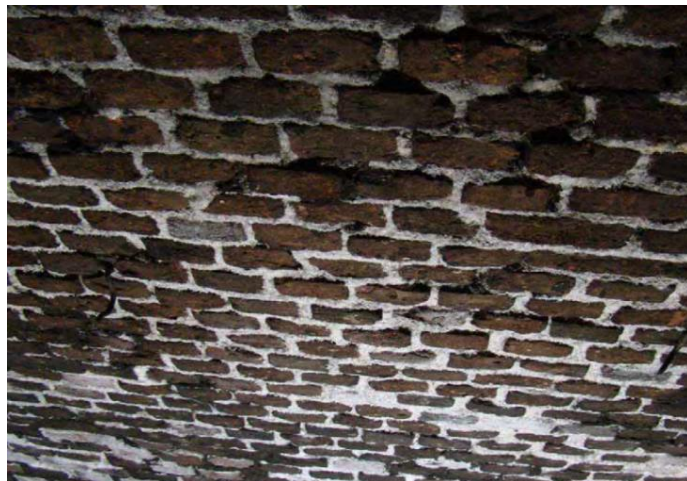
Figure II.9. Efflorescence en parement
