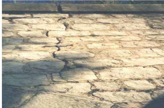
Figure II.15. Fissures de tympan
