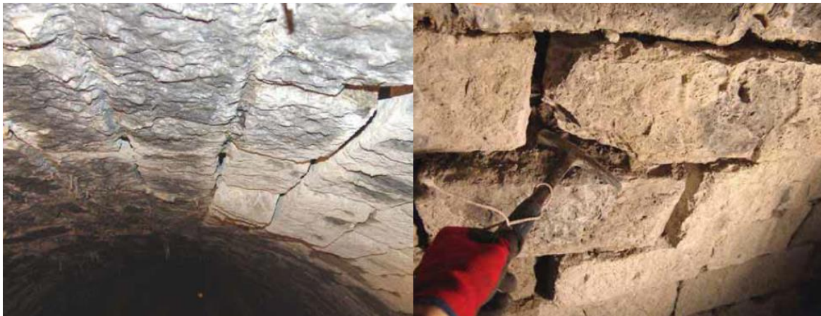
Figure II.7. Disjointement profond
