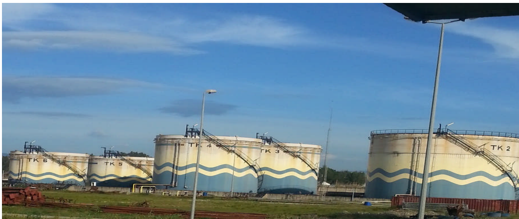
Figure I.1 : bacs de stockage carburants
