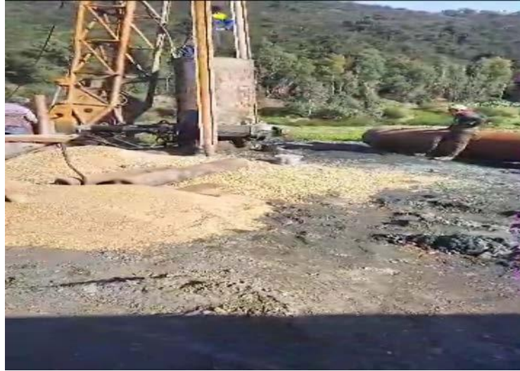
Figure 39 : Installation du tube guide (original)
