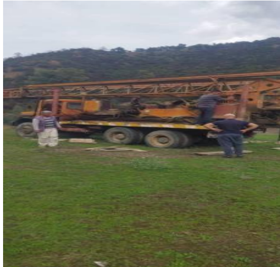
Figure 32 : Installation de la machine de battage (original)
