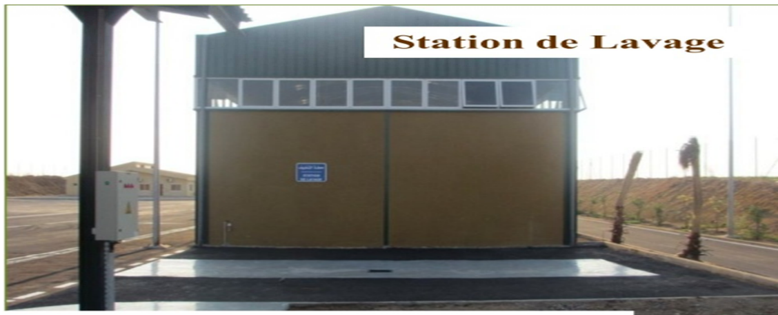
Figure N° 10 : Station de lavage
