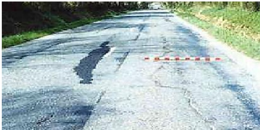
Figure 11.I. Fissuration d'adaptation.
