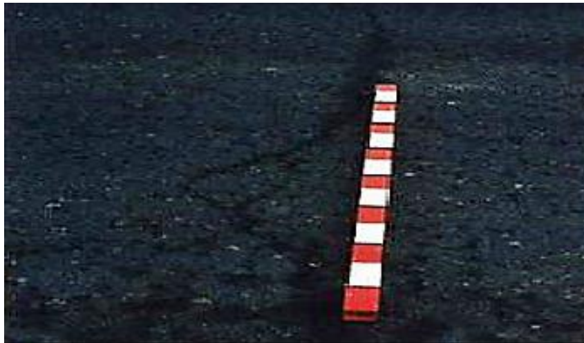
Figure 9.I. Fissuration transversale.
