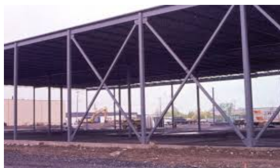
Figure 128. Contreventement en X. Source: http://searchguide.level3.com
