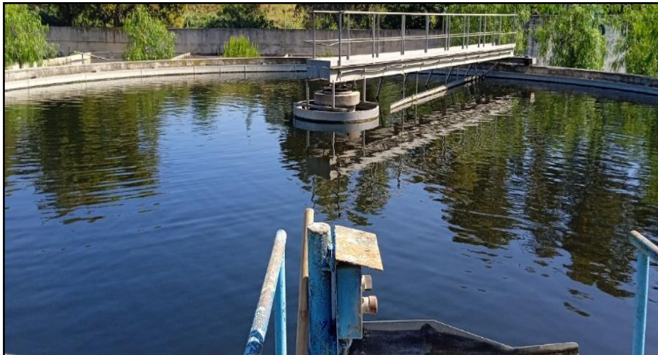
Figure 11 : bassin de clarification.
