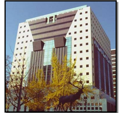
Fig.42: Public Services Building Michael Graves
