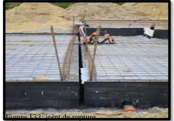
Figure 133: joint de rupture
