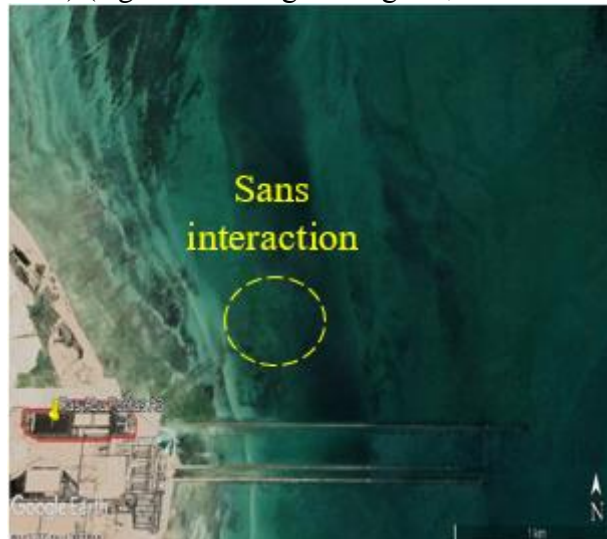
Figure II.14 : Image satellite de la station de dessalement Ras Abu Fontas A3 [31], [50].
