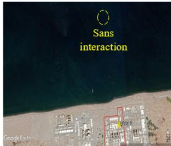
Figure II.12 : Image satellite de la station de dessalement Barka 2 [31], [50].
