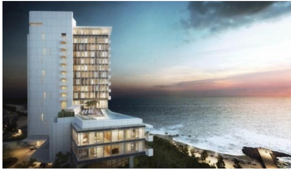
Figure 108 : 1 le bâtiment principal (la tour) Source: https://www.archdaily.com/781405/seamarq-hotel-richard-meier-and-partners .
