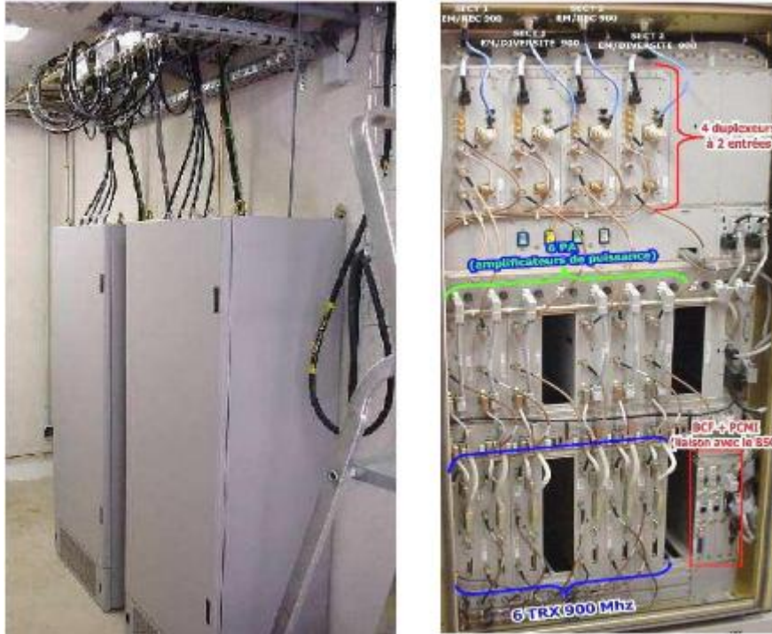
Figure I.8 : Station de Base BTS
