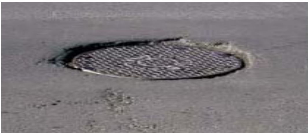
Figure 2.21. Dénivellation des regards
