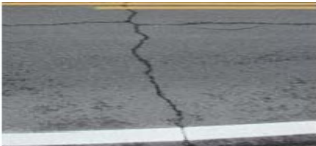
Figure 2.10. Fissure transversale
