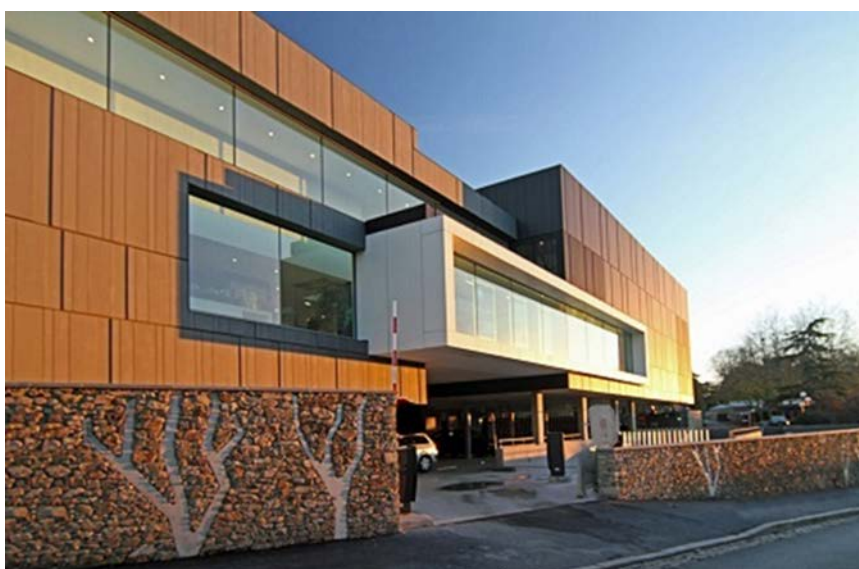
Figure 93 : le long court
