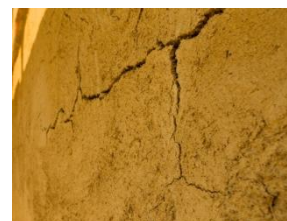
Figure 37 : Fissuration
