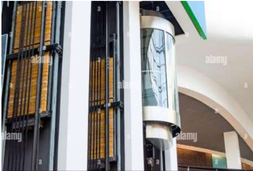
Figure 26: Les contrepoids
