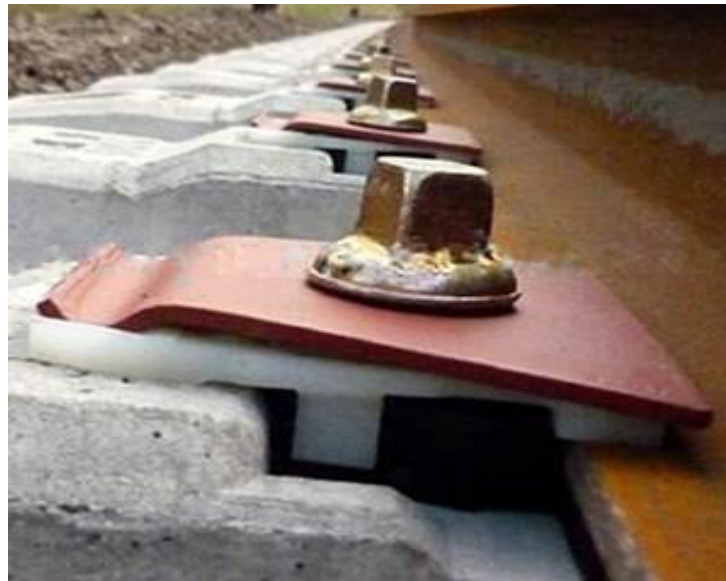
Figure VI-14: Attache de type Nabla.
