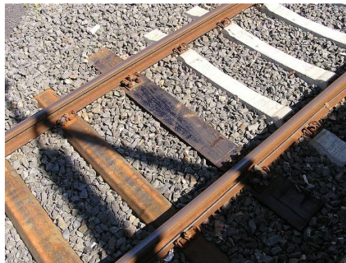
Figure VI-11: Traverse en acier.
