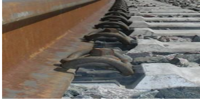
Figure VI-13 : Attache de type Vosloh.
