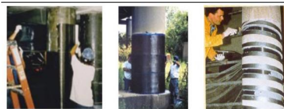
Figure II.15 : Stratification au contact (WBAC 2003) [43].
