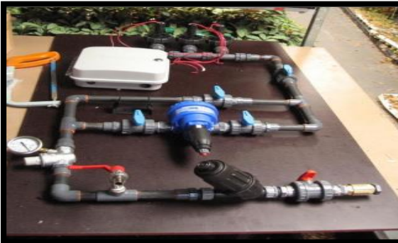
Raccordement de la station d'irrigation
