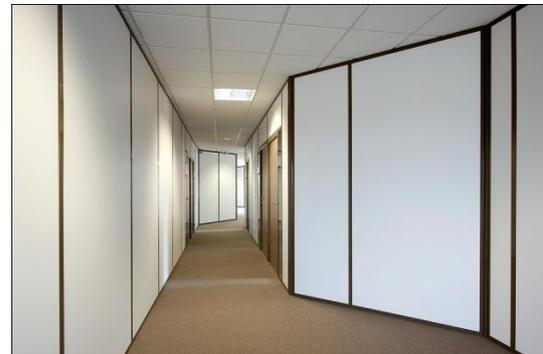
Figure 9: Cloison plaque de plâtre.
