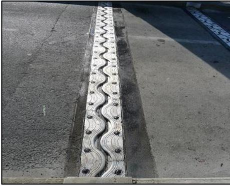
Figure 4 Joint sismique
