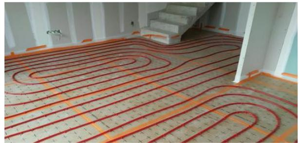
**Figure 169:** plancher chauffant, source :[https://conseils.xpair.com/agenda\\_news/plancher-chauffant-rafraichissant-marche-croissance.htm](https://conseils.xpair.com/agenda_news/plancher-chauffant-rafraichissant-marche-croissance.htm)
