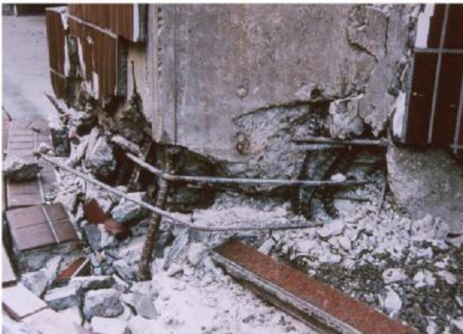
Figure IV.36 Plastic ball joint at the base of BA post
