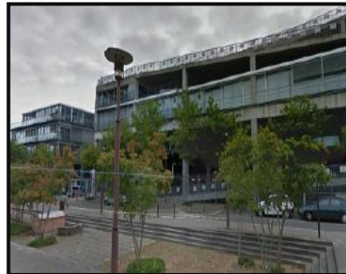
Figure 178: L'ENSA de Nantes Source : https://www.amc-archi.com/article/ecole-nationale-superieure-d-architecture-nantes.16823
