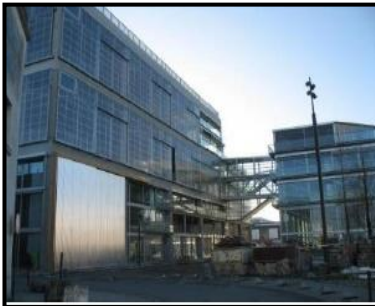
Figure 179: L'ENSA de Nantes Source : https://www.amc-archi.com/article/ecole-nationale-superieure-d-architecture-nantes.16823
