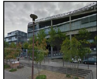
Figure 177; L'ENSA de NANTES Source : https://www.amc-archi.com/article/ecole-nationale-superieure-d-architecture-nantes.16823
