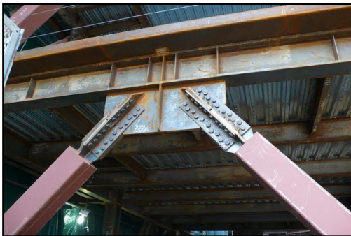
Figure 200: Assemblage poteau incliné/ poutre métallique Source : https://i0.wp.com/www.southernsteelengineers.com/wp-content/uploads/2019/02/Seismic-Chevron-Connection-1.jpg?fit=1404%2C788&ssl=1
