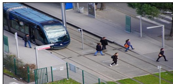
Figure 92: Station de tramway interne Source : https://operation-campus.u-bordeaux.fr/Agir-pour-un-campus-durable/Mobilite .
