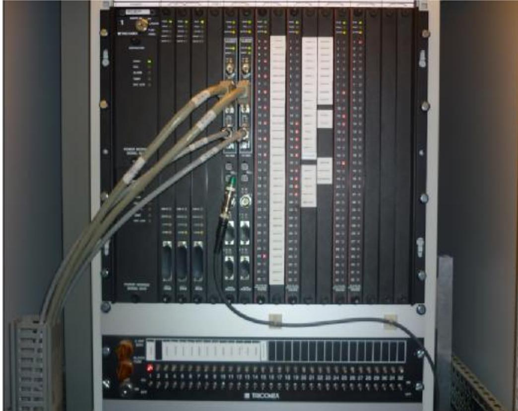
**Figure III.1 : Automate programmable (TRICONEX)**
