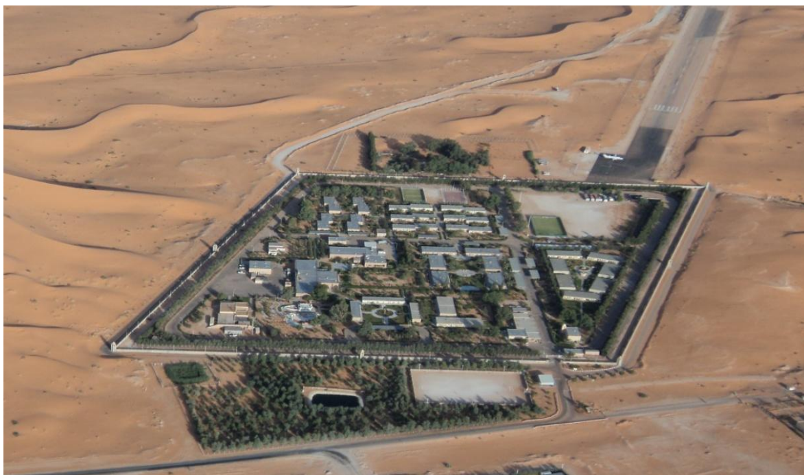
Figure 14 : site BRN base de vie
