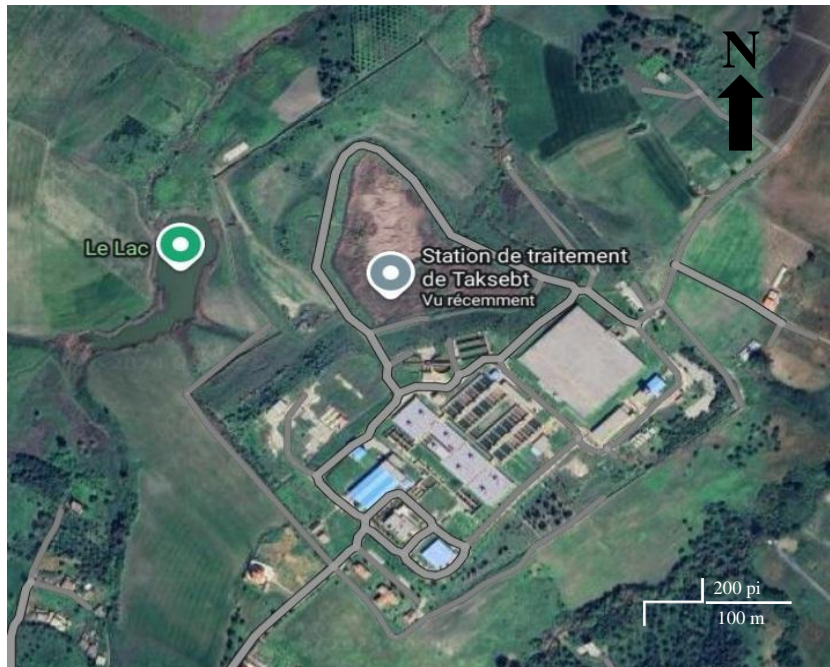
Station de traitement Taksebt Tizi-Ouzou (source : Google Maps)
